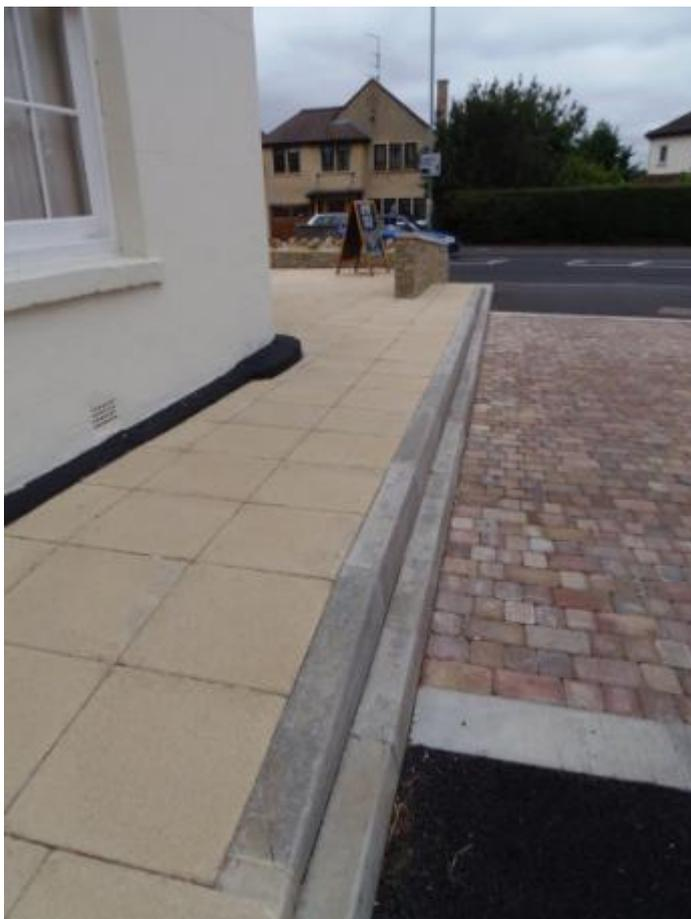
**Figure 8** Confusing change in gradients on the hotel side pavement
