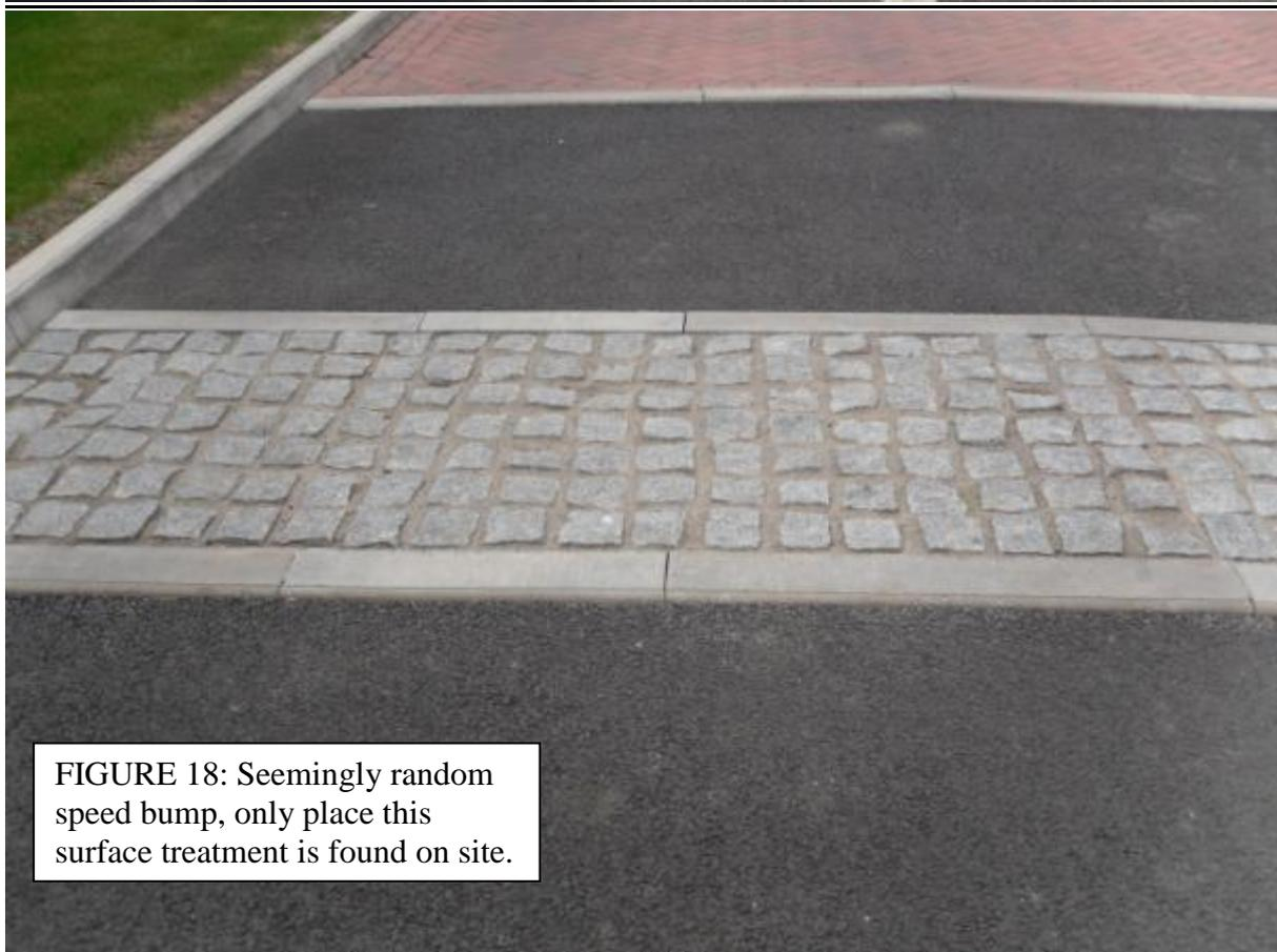
FIGURE 18: Seemingly random speed bump, only place this surface treatment is found on site.
