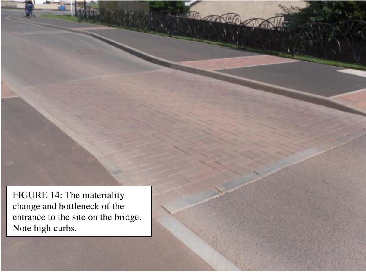
FIGURE 14: The materiality change and bottleneck of the entrance to the site on the bridge. Note high curbs.
